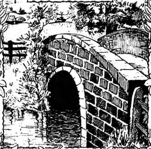
THE OLD BRIDGE OVER THE RYLL NEAR ST JIMS
